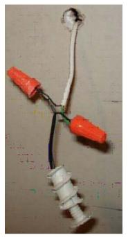
FIG. 15 Sensor wire connected to cable
